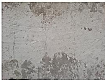
(a) Early Shrinkage Cracking
