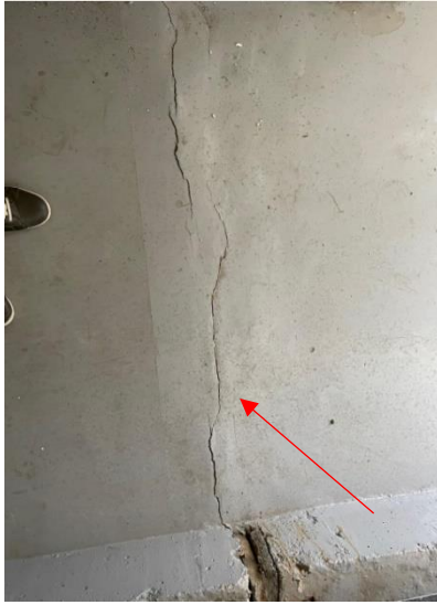
a) Surface crack appearing along expansion joint
