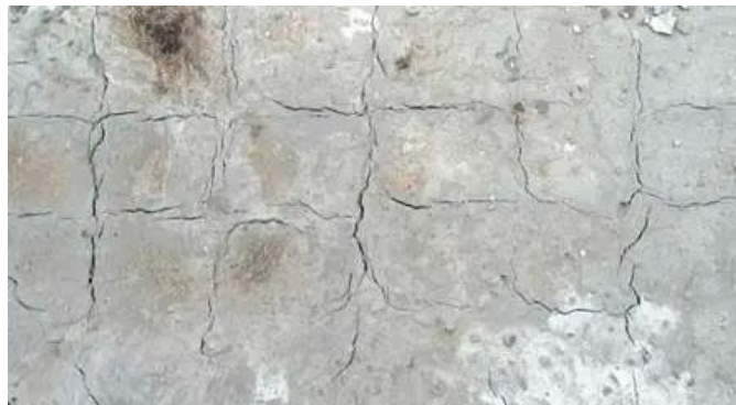
Figure 1 Shrinkage cracks in Slab [5]
