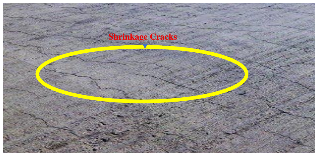
Figure 1. Visible shrinkage cracks reduce structural integrity of pavement due to moisture infiltration.
