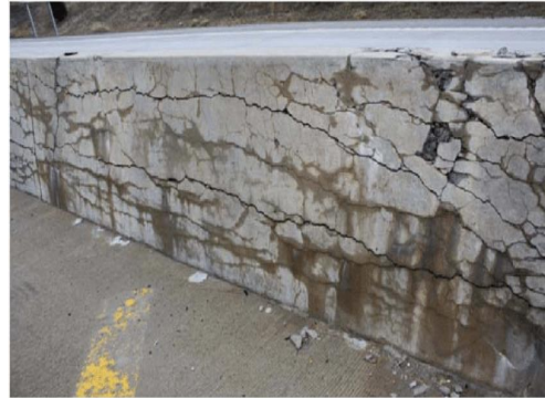
Figure 1. shows the overpasses that are crucial parts of our transportation infrastructure, ensuring safe passage for vehicles and pedestrians. Regular Alkali-Silica Reaction (ASR) testing and prevention measures are essential to maintain their safety and longevity [8].
