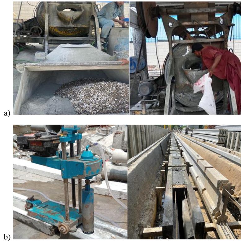
Figure 2: (a) Material mixing in the concrete mixer (b) placement of concrete in the shuttering bed and cores taken out from prestressed beams
