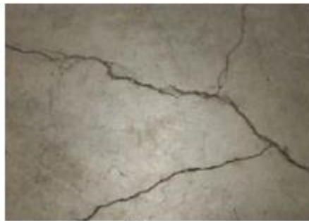
Figure 1: Presence of flexural cracks in slab Mydin [33]
