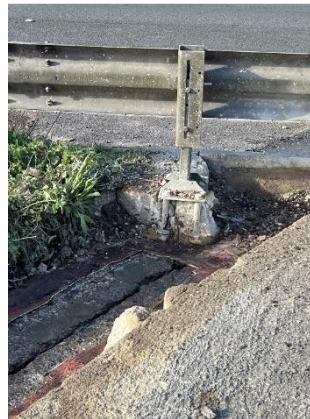
Figure 5: Presence of a vehicle restraint system post at expansion joint location.
