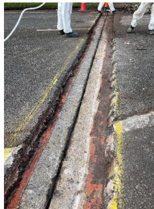
Figure 4: Existing bridge waterproofing left in place to provide lapping with new waterproofing system to be installed at buried joint.
