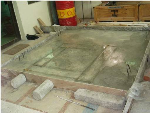
Figure 4. Complete concrete pad being cured
