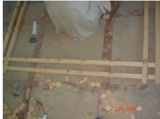
Figure 5. Rectangular skeleton of timber elements
