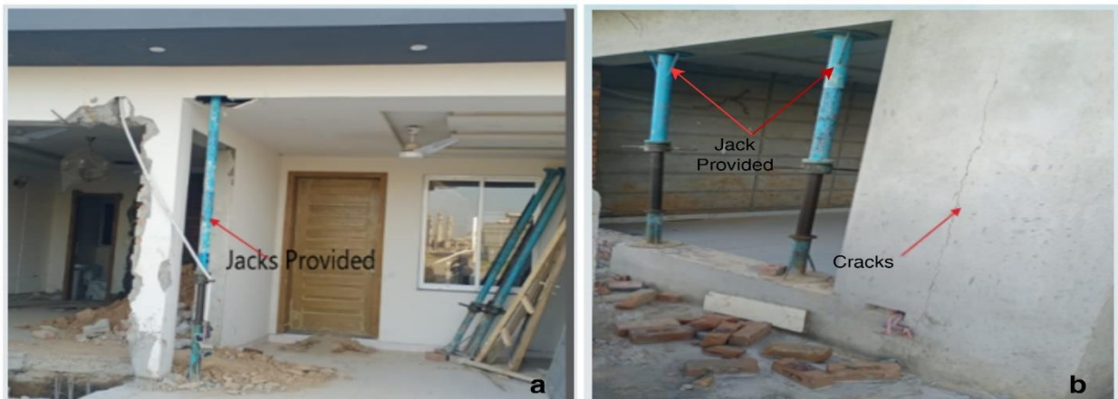
Figure 1:(a,b) Jacks are used to prevent settling in both freshly built and older homes, as well as fissures caused by expansive soils' volume change behaviour .
