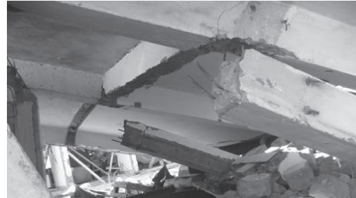
Figure 4: Anchorage failure [1]
