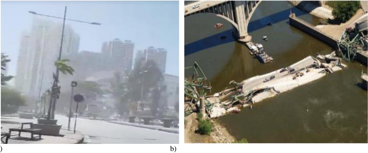
Figure 3: a. wind and sandstorm event happened at Gurney [25] and b. collapsed bridge center section [28]
