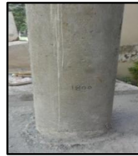
Figure 5. Grinded and Prepared surface of pier for CFRP application.
