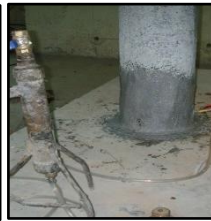
Figure 4. Outer repair works with cementitious mix after filling of cracks
