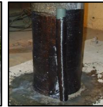
Figure 6. Application of CFRP (HEX-103-C) to pier.
