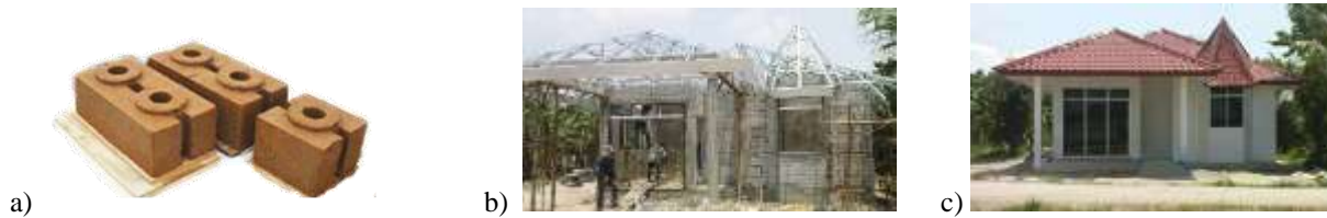
Figure 3: a. Innovation material interlocking blocks b. House construction using innovative material c. Sustainable house.
