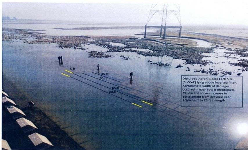
Figure 2: View of settled concrete blocks right under-sluice
