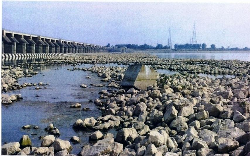
Figure 1: Dislodged concrete block carried away by river current in Front of Bay 51
