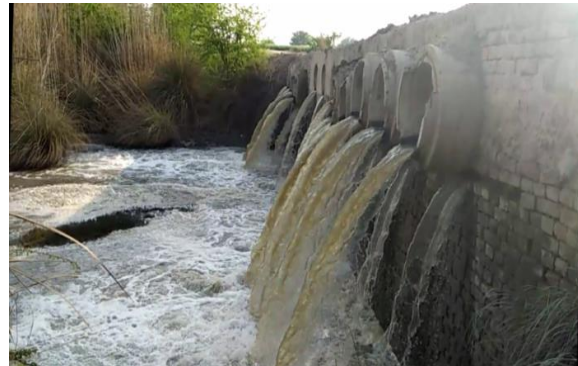
Figure 4: Combine (Feed + Mill + Injecting ) water discharging from Mill
