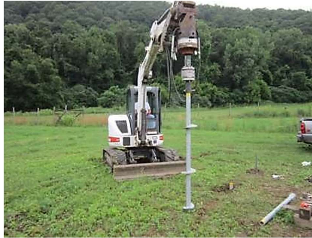
Figure 2: Drilling of Helical Pile [16].
