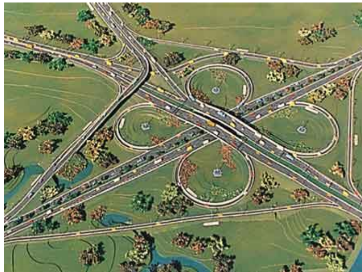
Figure 1: Aerial view of Faizabad Interchange showing the clover leaf, the overhead, and the underpass.
