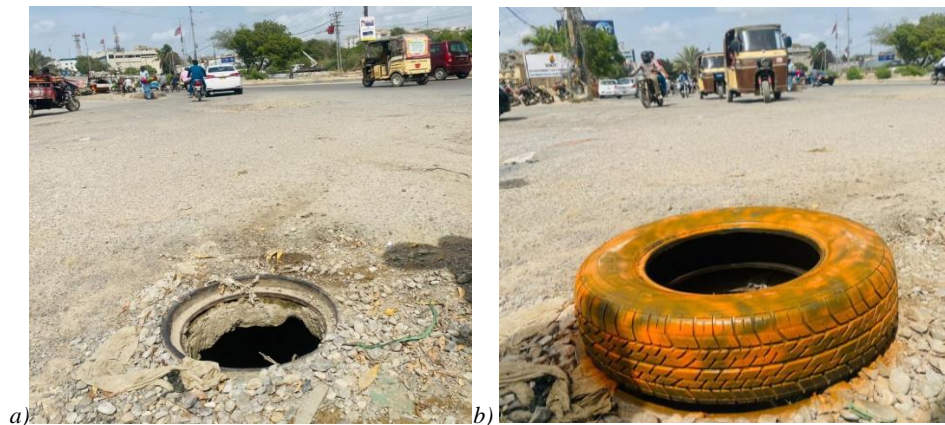
Figure 3: a) before the installation of rubber tire, b) after the installation of rubber tire.
