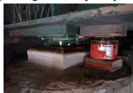
Figure 2: Hydraulic jack placed on column with limited space
