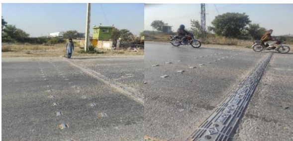
Figure 1: Steel speed hump along with Road studs
