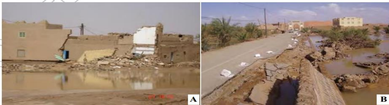
Figure 7 A & B: Destroyed Houses, Roads and water Supply lines [23]
