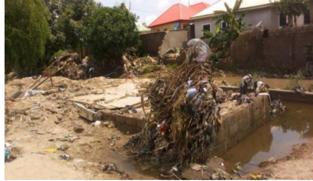
Figure 5 b: Completely Destroyed Building [12]
