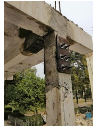
Figure 2-4: Through Anchorage in beam
