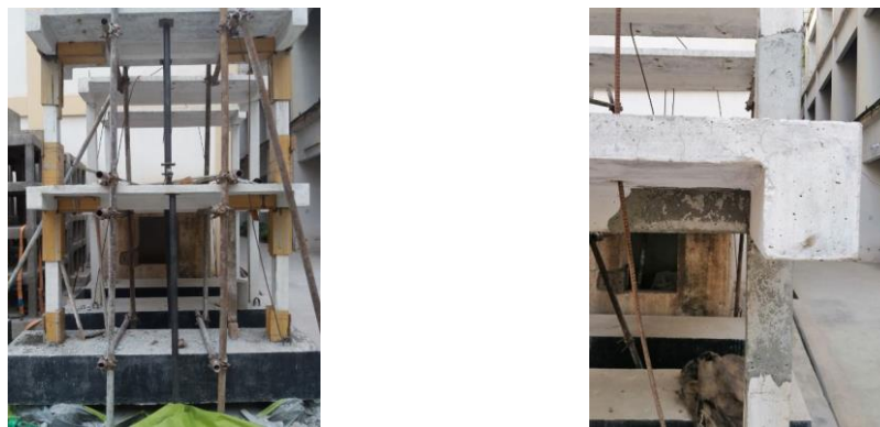
(d) Formwork for concreting, (e) Joint after replacing damaged concrete
