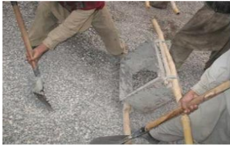
Figure Error! No text of specified style in document.-1: Manual batching and mixing
