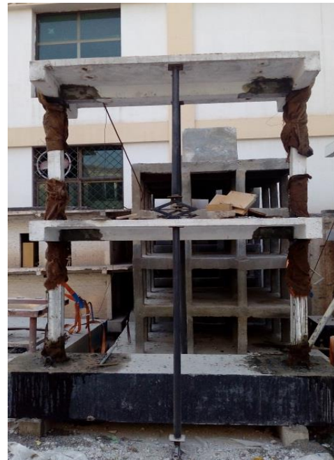
Figure 2: Removal of damaged concrete. Figure 3: Replacement with rich concrete.
