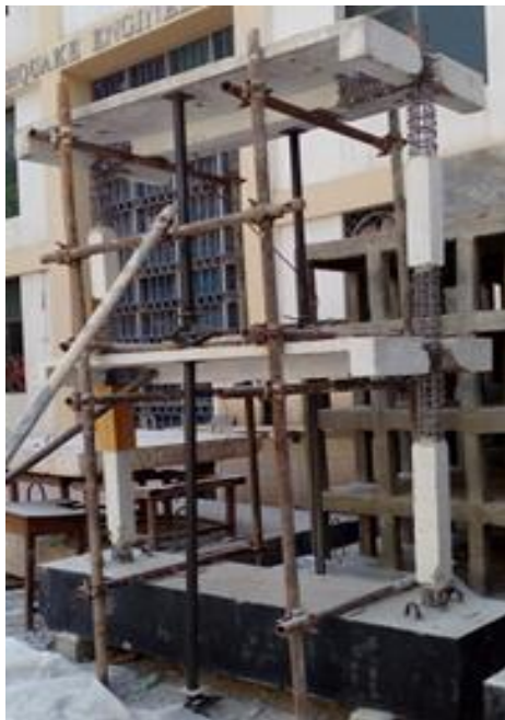
Figure 2: Removal of damaged concrete. Figure 3: Replacement with rich concrete.
