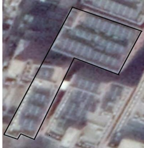
Figure 1: Aerial view of buildings
