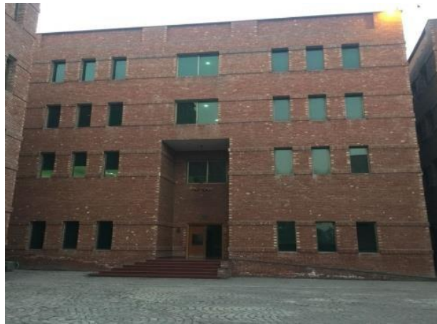
Figure 2: Front view of building
